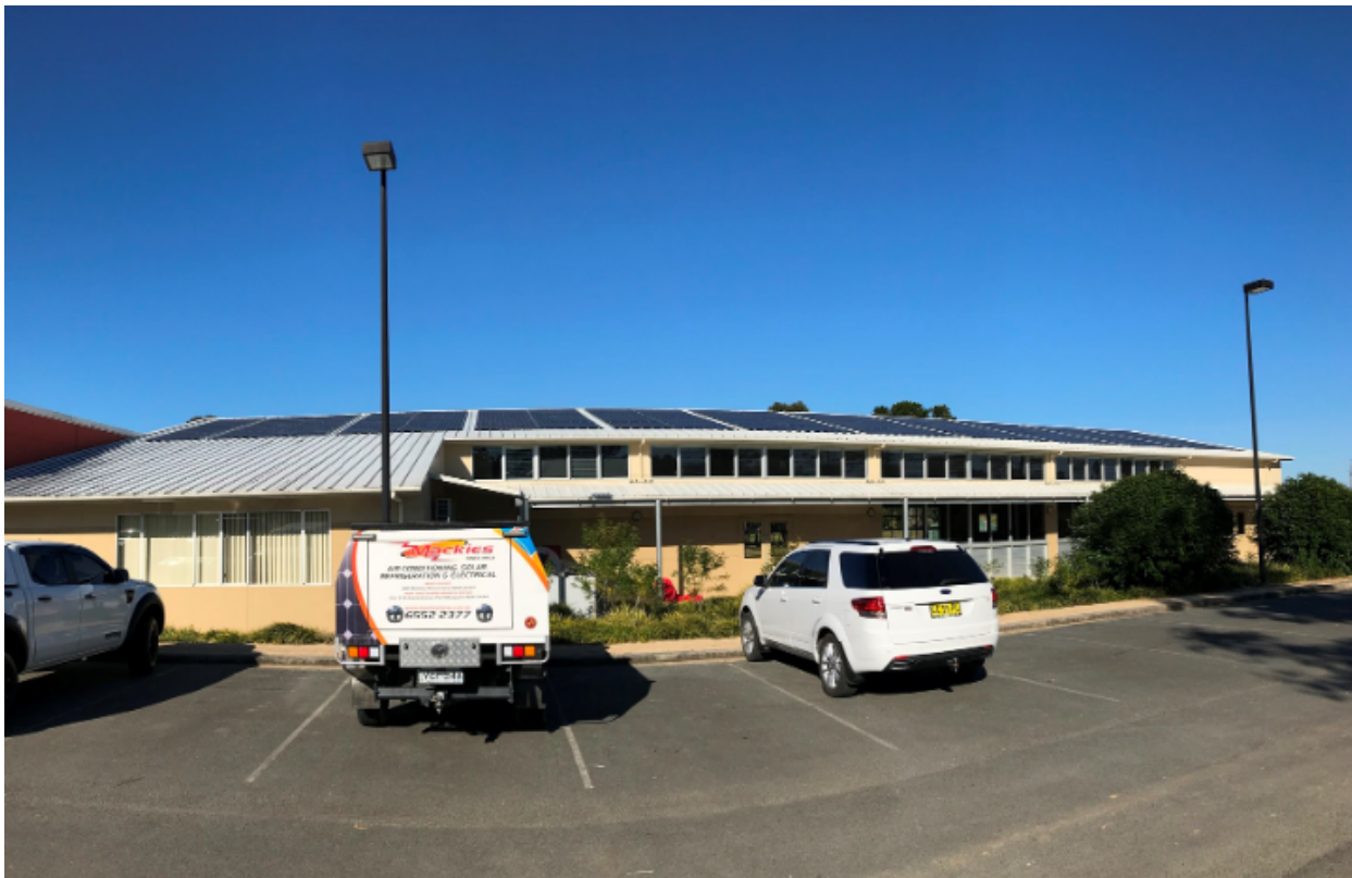
Mid north coast NSW - 60kw installed July 2018
