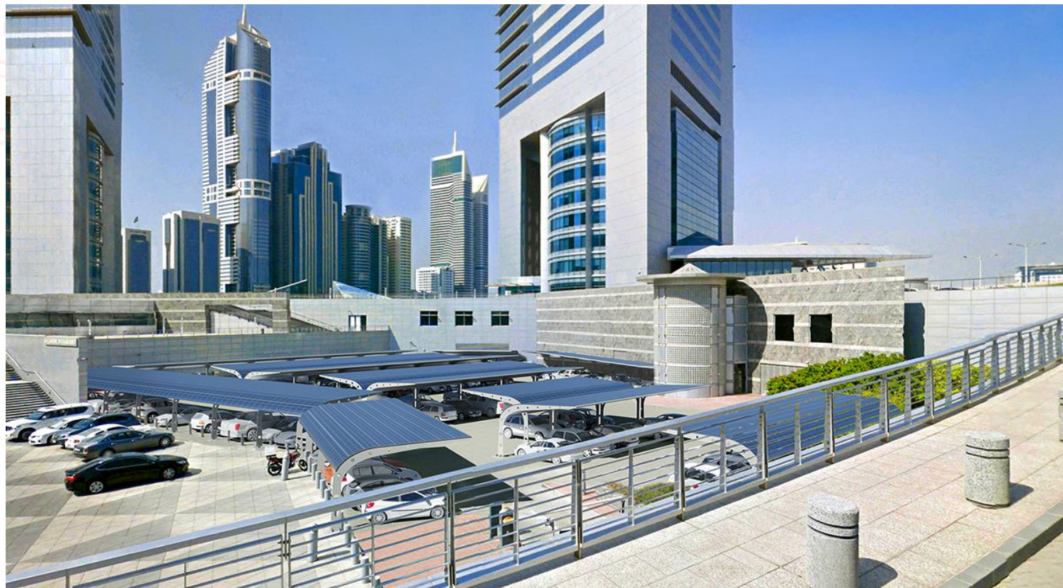
273 kw eArche – the Emirates Towers solar carport– Dubai, UAE
